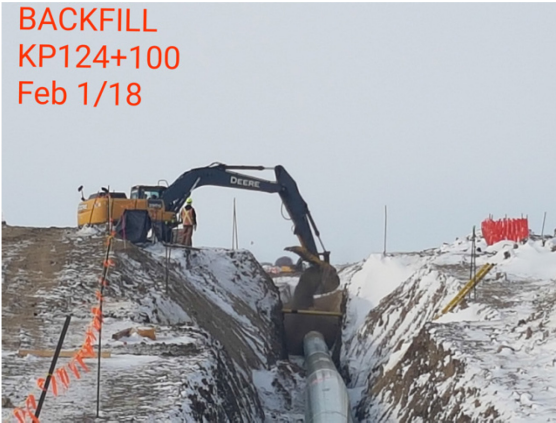
7. Backfill – Km 124+100 – Feb 1, 2018
