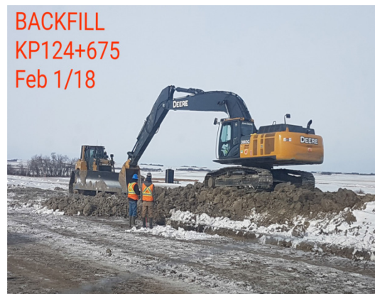
6. Backfill – km 124+675 – Feb 1, 2018
