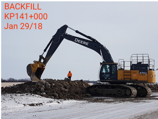
1. Backfill- Km 141+000 – Jan 29, 2018
