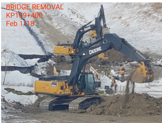
5. Bridge removal – Km 109+400 – Feb 1, 2018
